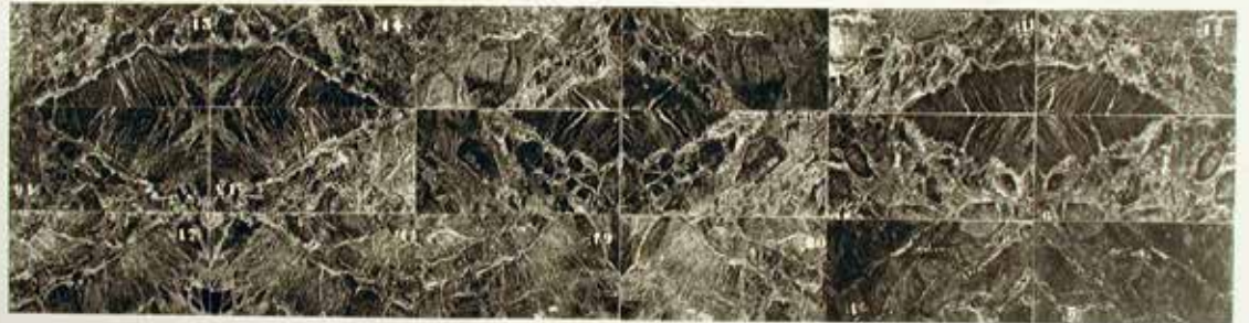
Fig. 25. Study for the positioning of the slabs of green marble on the wall over the interior pool.
